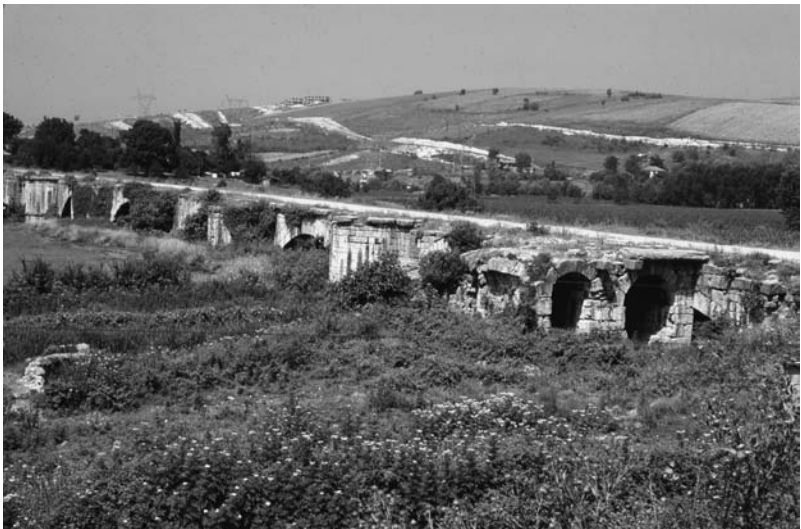
Fig. 1.29 Justinian's bridge over the Sangarius
